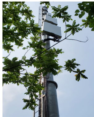
Figure 3: Galtronics temporary multibeam deployment at F1 in Montreal.
